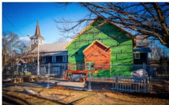
New Construction at Holy Redeemer - 2023
