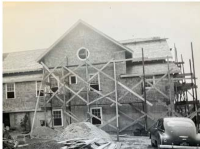
Early Renovation - 1950s
